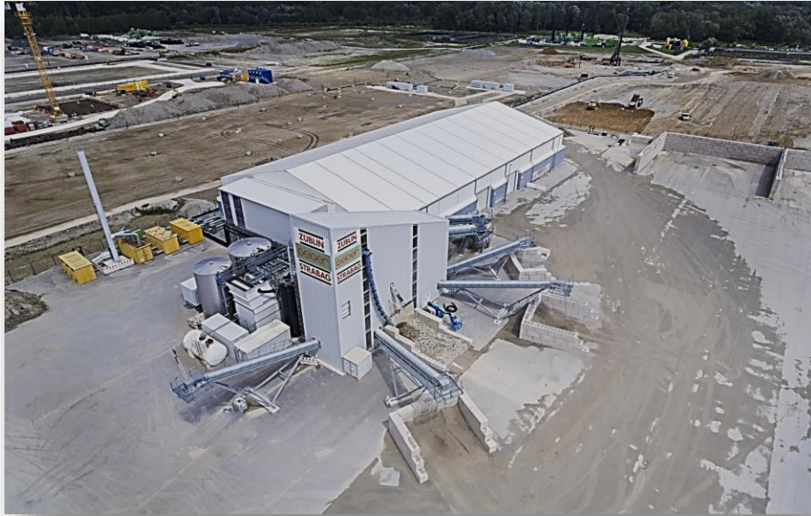
Figure 2.3- Areal view of the soil washing plant (front), sludge treatment facility (left hand side) and the reception hall (in the back). Copyright: ARGE AUDI IN-Campus GbR (ask for permission to Dr. Benjamin Faigle – Züblin Umwelttechnik GmbH)
