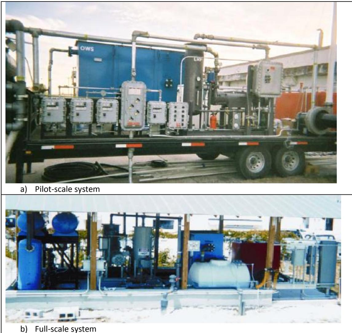
Figure 2.6.: Installed and operated bioslurper system [5]
