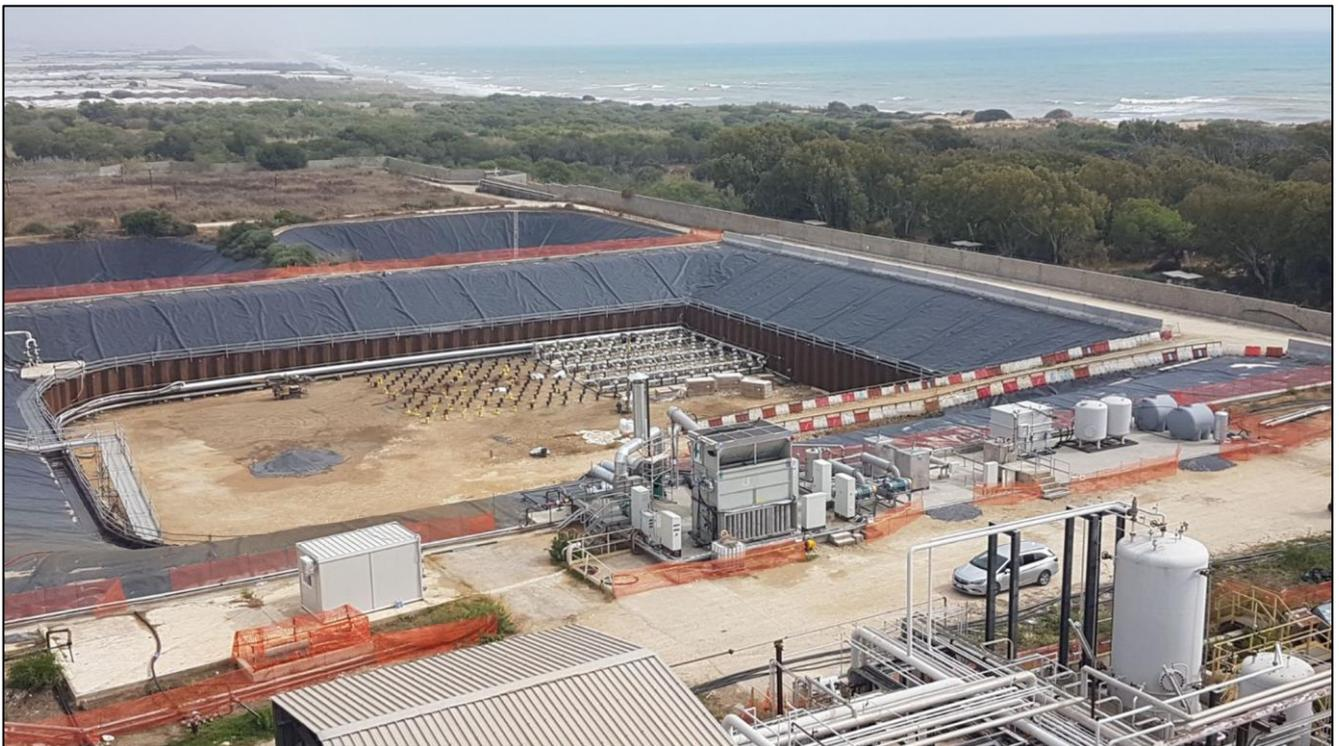
**Site view, during the intervention phase with the installation of remediation systems (see Chapter 4) and Vapour Treatment Unit (upper edge of the basin).**
