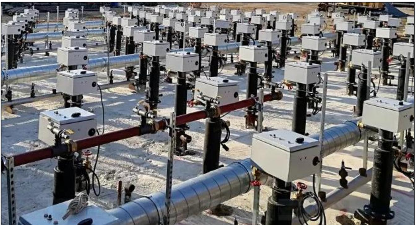
During the heating and for the entire treatment period, the contaminants, in gas phase, are extracted by steam extraction probes, positioned in the soil, near the heating points, to then be conveyed inside stainless steel pipes and sent to the vapour treatment unit. General scheme of remediation project is in the following page.
