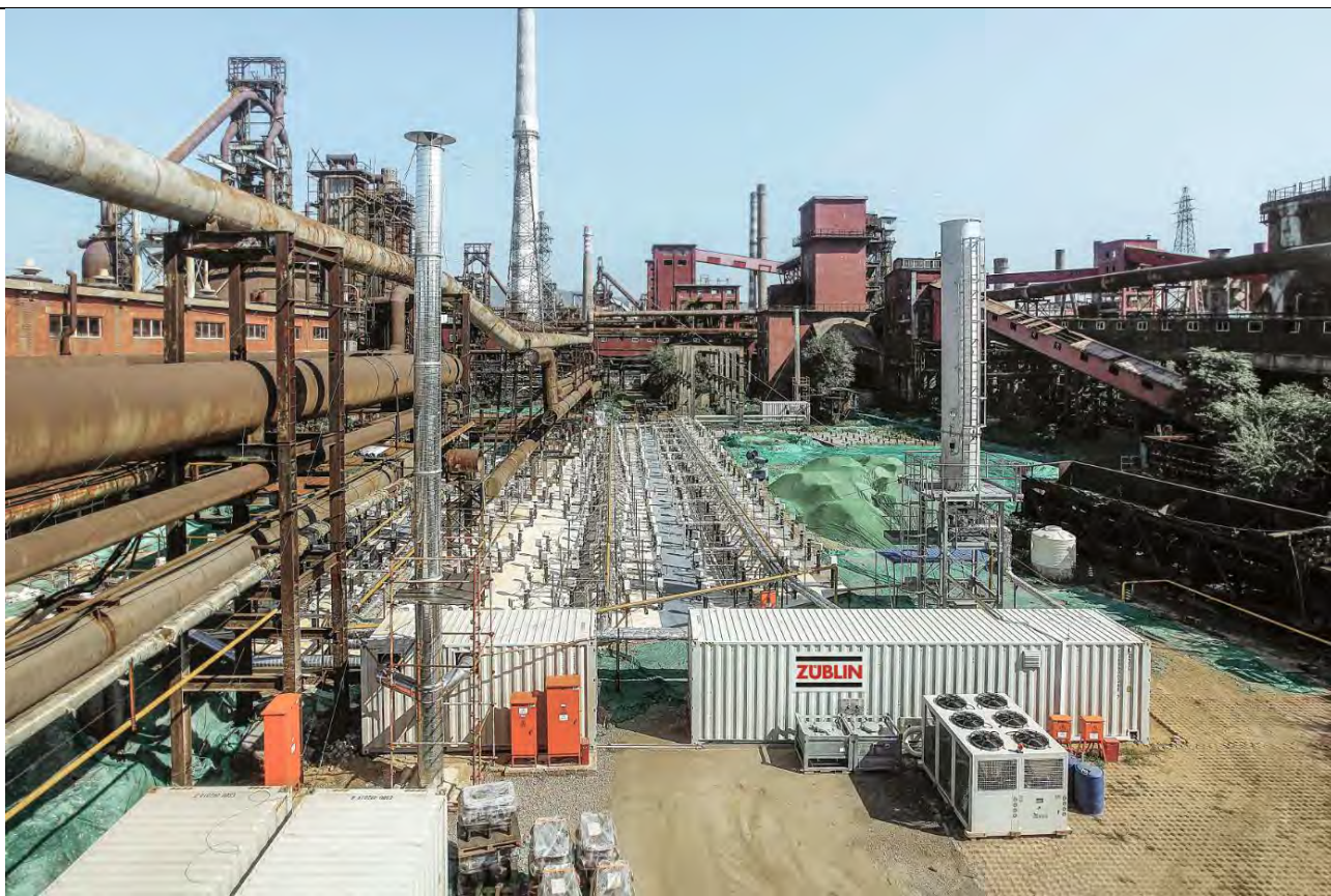
Figure 14 - Heating elements and treatment plants in ISTR-area 4
