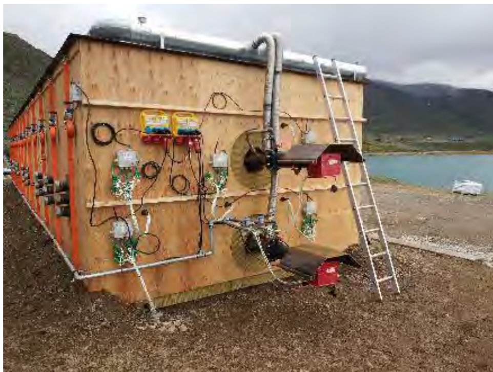
Figure 4 – Container on site (back)
