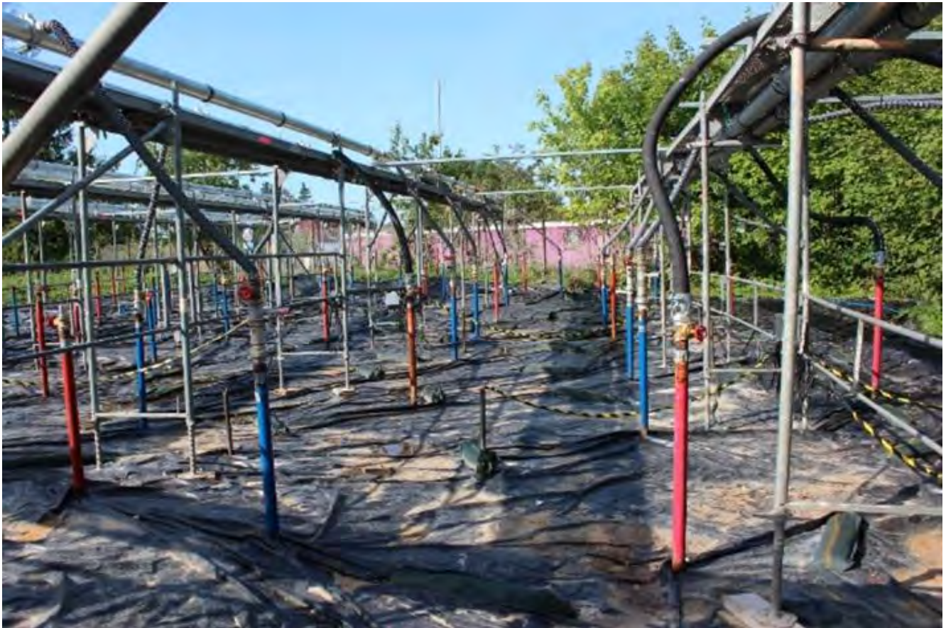
Fig. 8: Development of remediation area (red = injection well, blue = extraction well)
