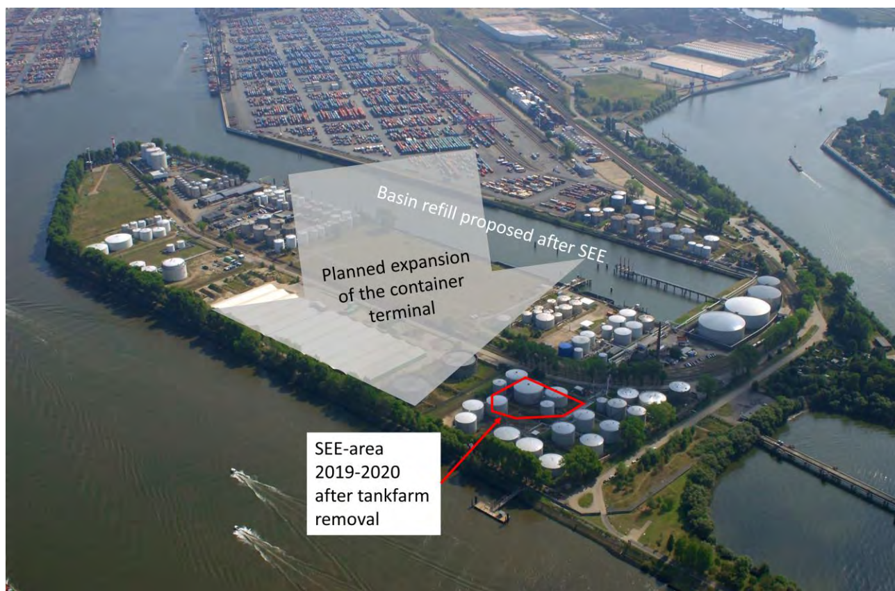
Figure 2 – Hamburg Petroleum Port: Petroleum tank farm (in the period 2000-2010), location of SEE treatment target zone in red (2019-2020, red marked area) and proposed project development (from 2021).
