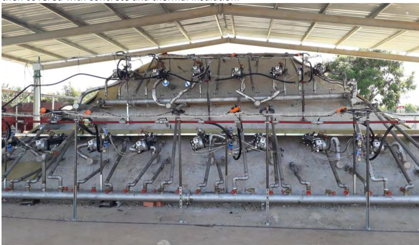
Figure 3 – Front picture of the pile on site
