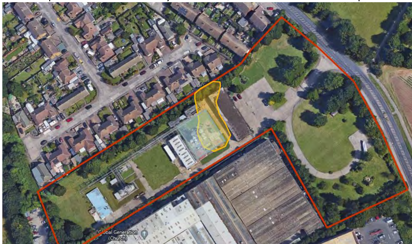
Figure 1 – Site view from above
