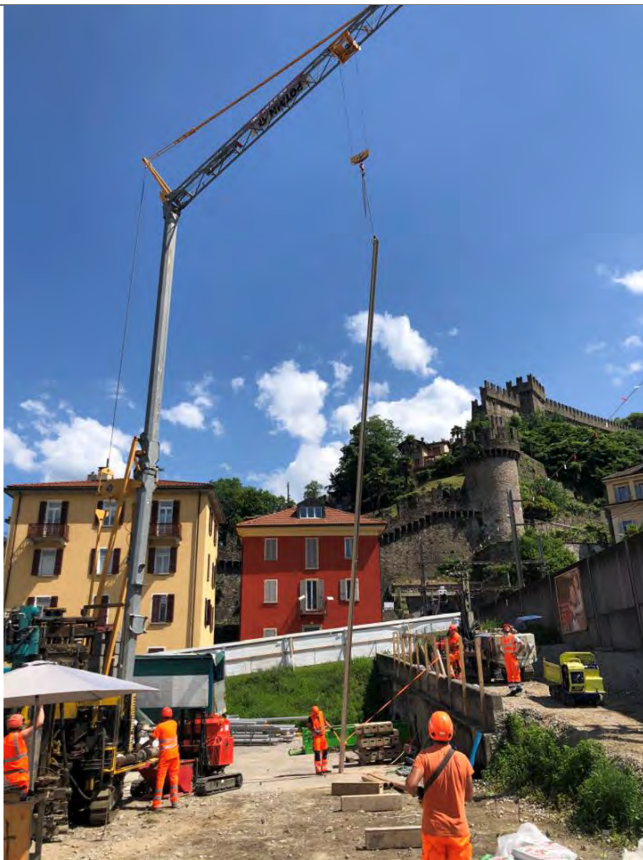
Figure 11 - Erecting a protective tube with the help of a tower crane near the railway tracks
