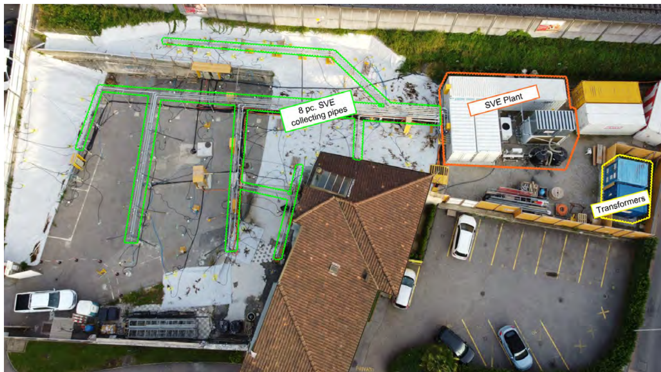
Fig. 14: Drone shot of the remediation area with SVE plant and transformers (right)
