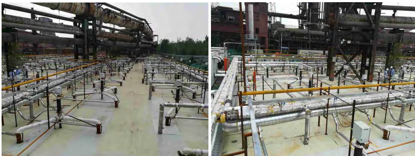
Fig. 15 - Heating elements and treatment plants in ISTR-area 5
