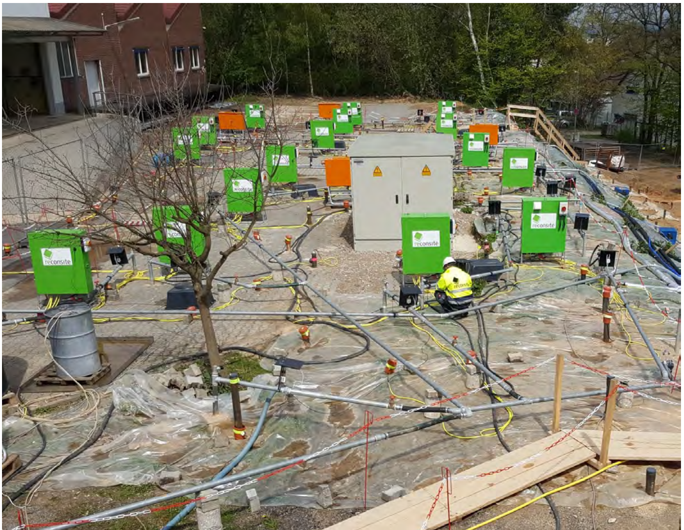
Figure 4 - View of the in-situ thermal remediation TTZ (field 1) using the THERIS method (electrical driven heater wells).
