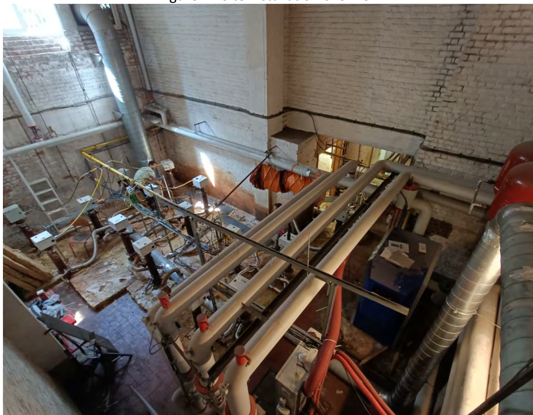
Figure 5 - One of the cellars of the site
