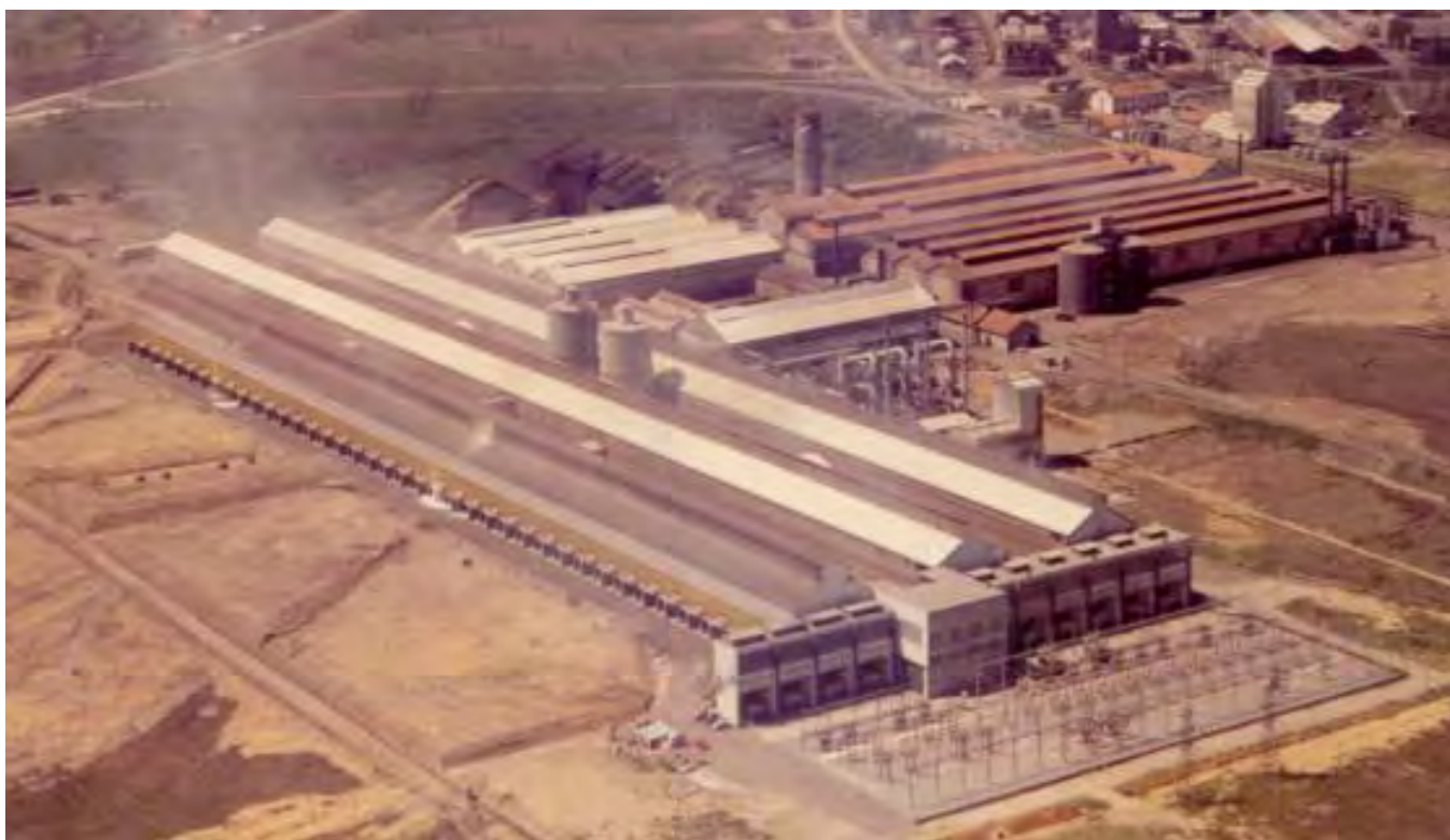
Figure 1 - View of the former factory; circled zone shows the electrical substation and 2 high voltage line in the bottom.
