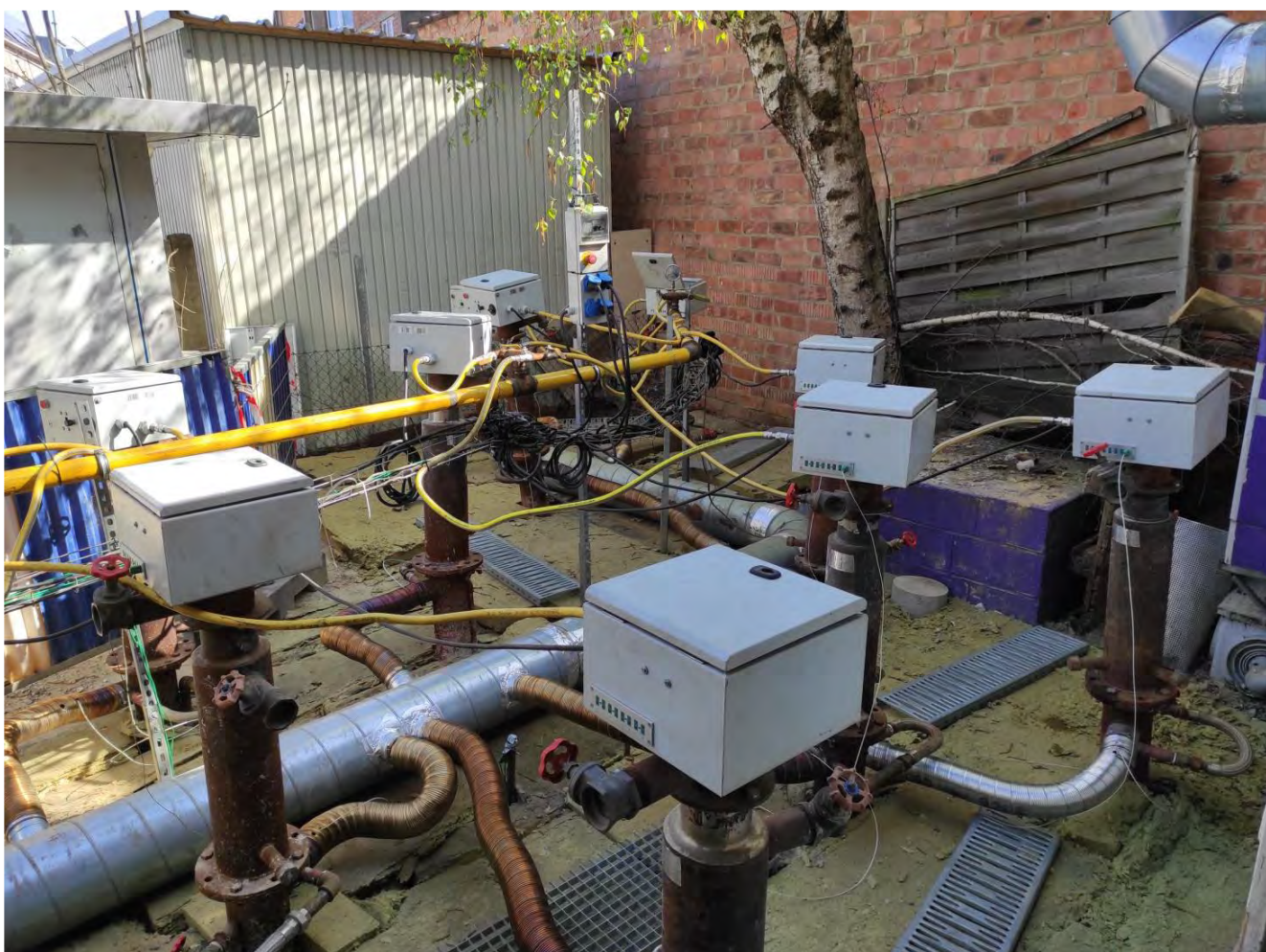
Figure 3 – Treatment Zone 1 in the outside yard
