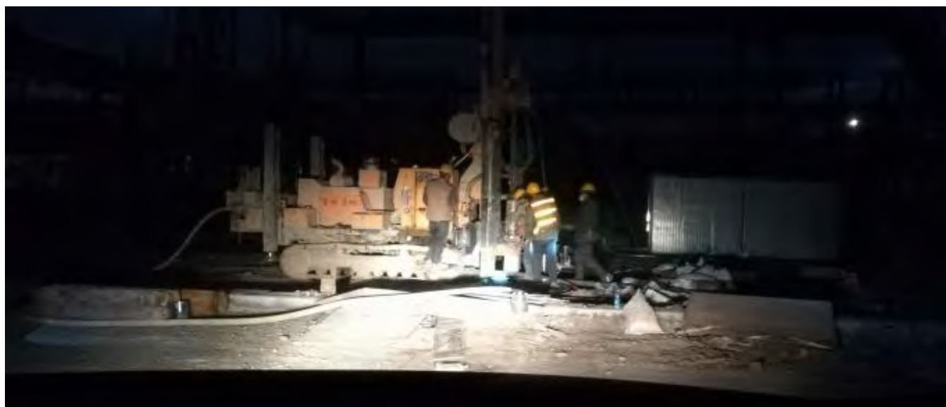
Fig. 18 - Drilling works during night shift
