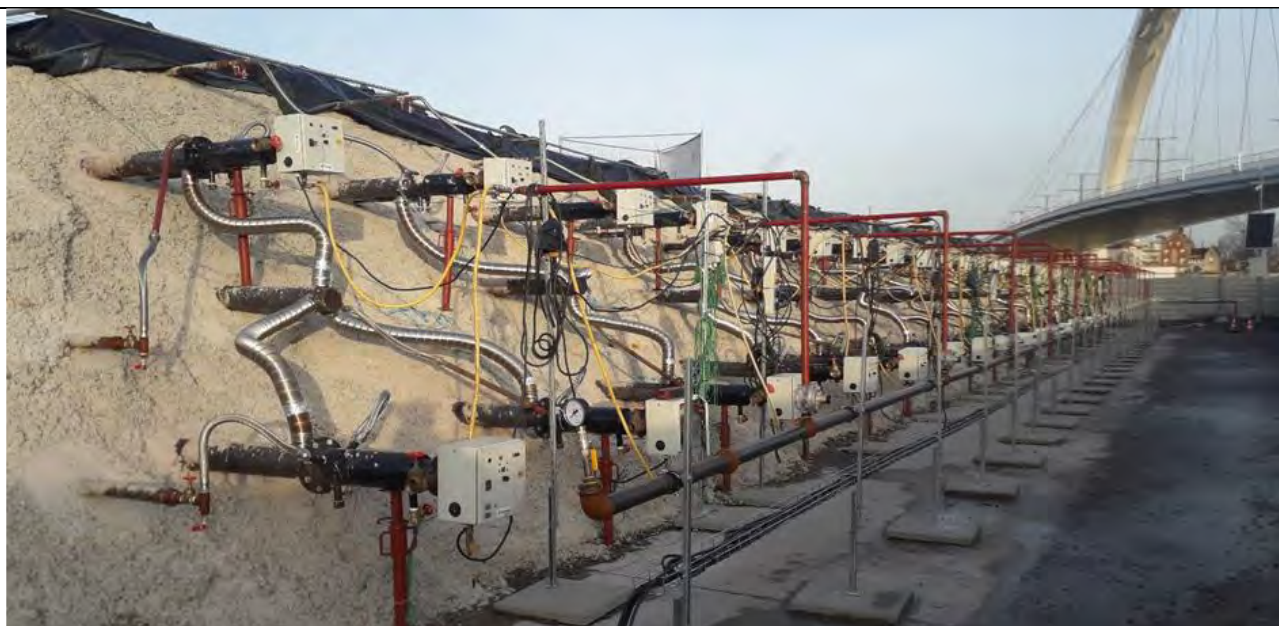
Figure 4 – ESTD installation on site
