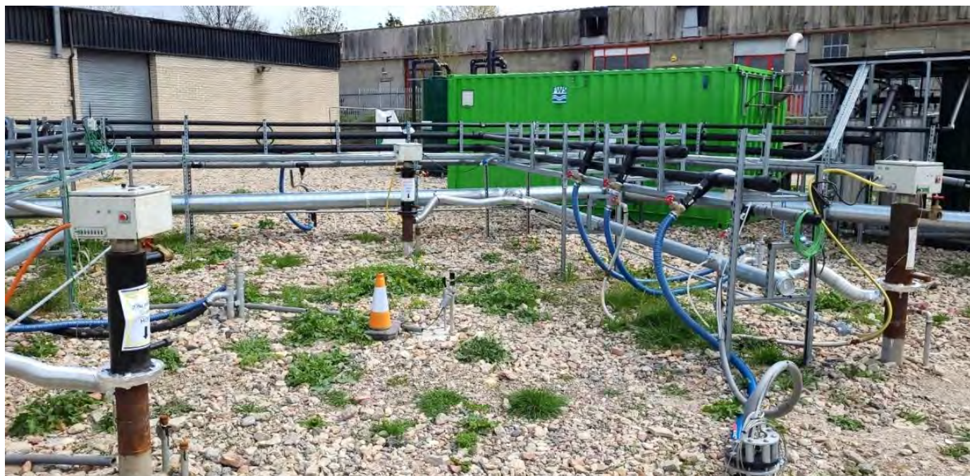
Figure 2 – ISTD installation on site
