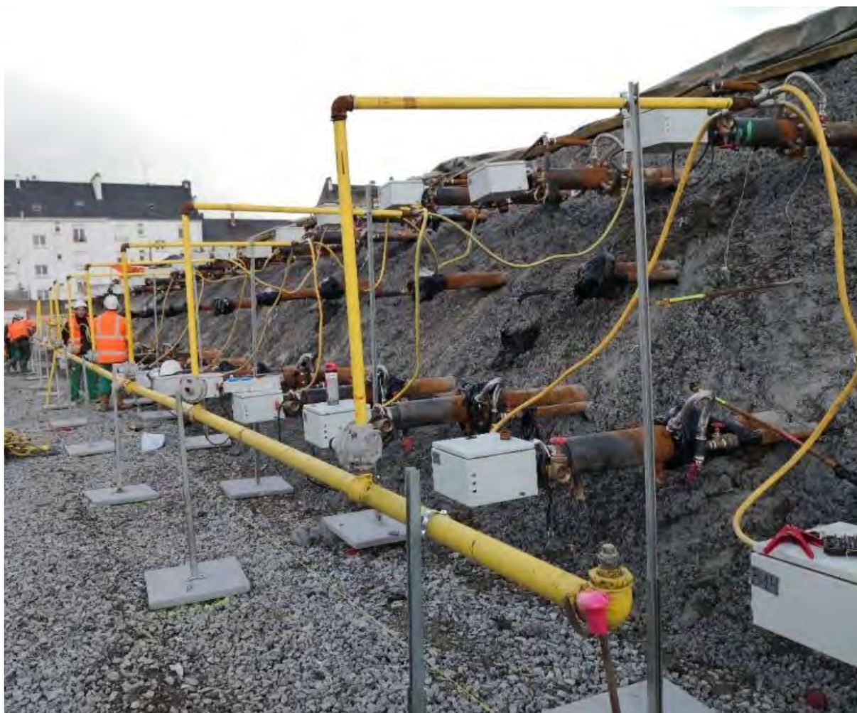
Figure 2 – Gas network and burner's distribution
