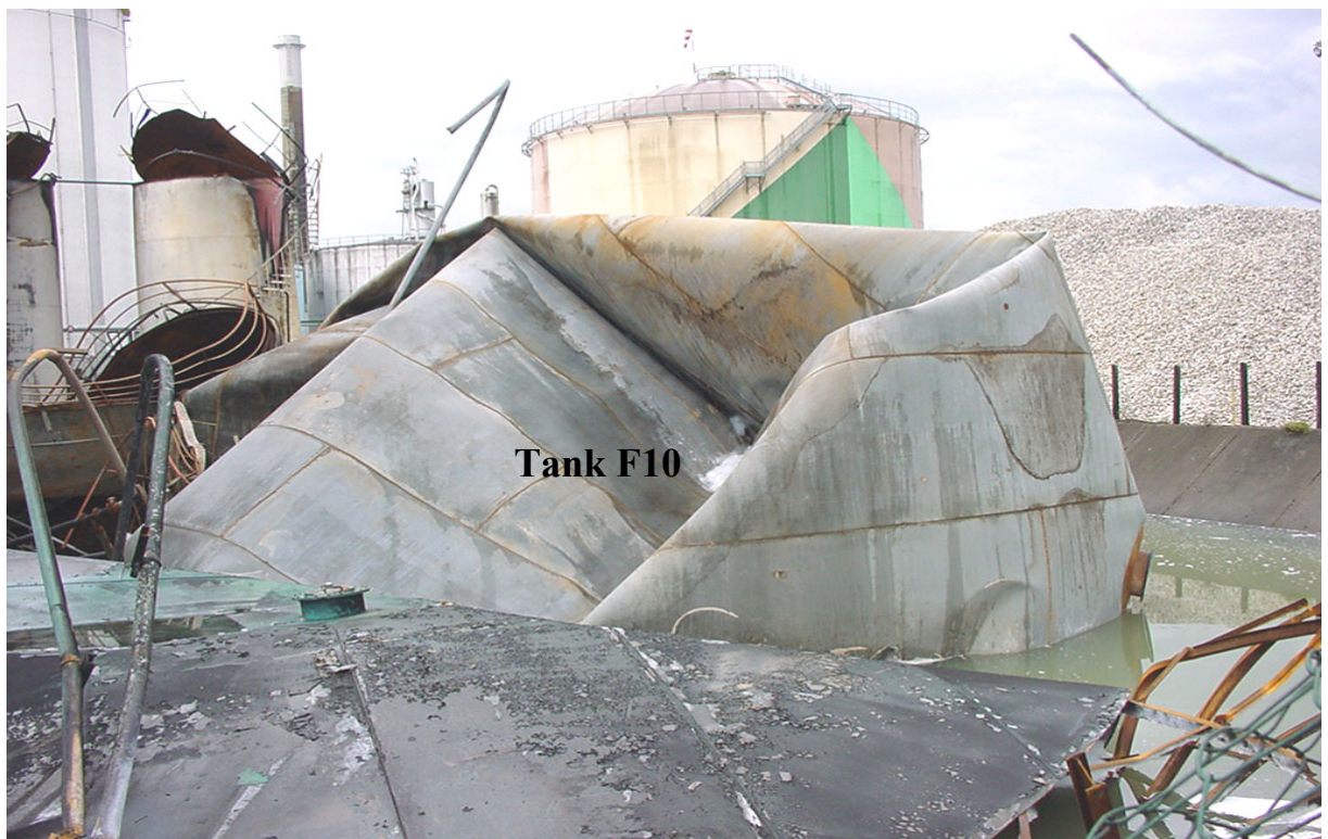
Roof of tank F10
