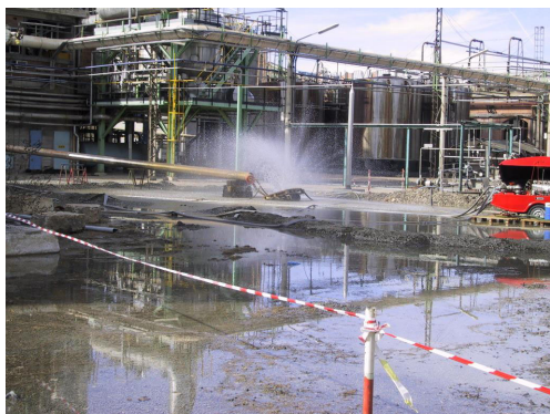
Dilution of NH 3 by water curtains
