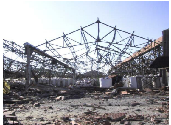
Warehouse destroyed by the explosion
