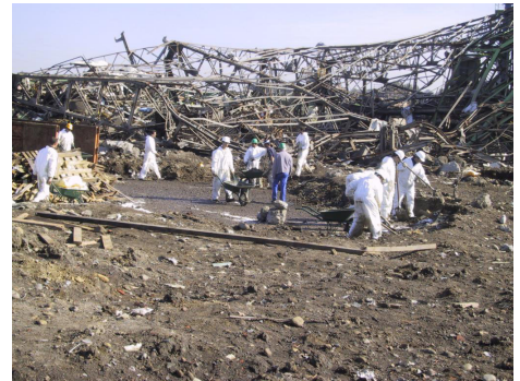
Site clean-up operations
