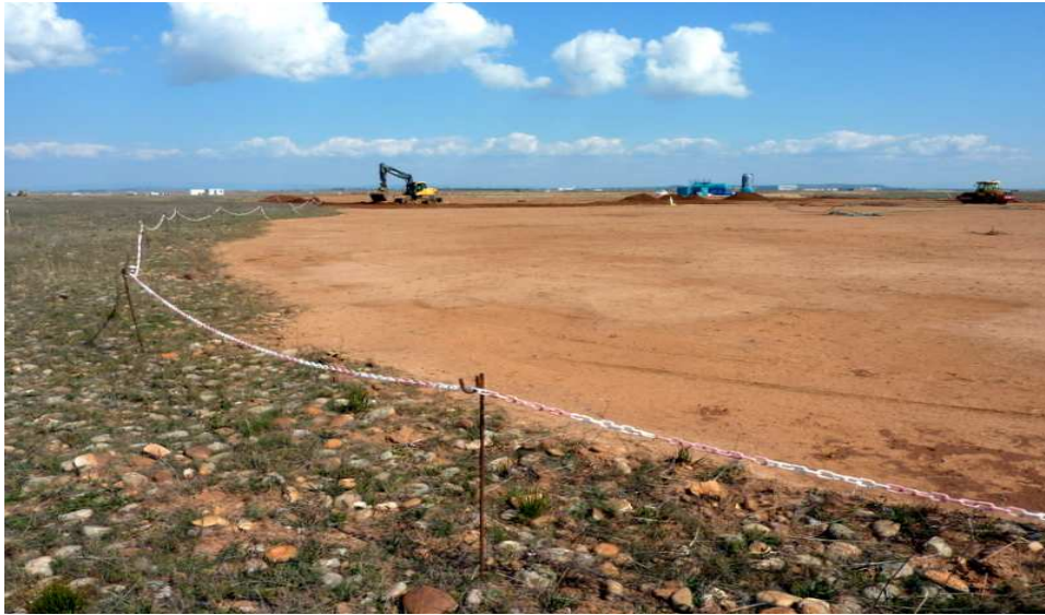
Restored and compacted zone - RR
