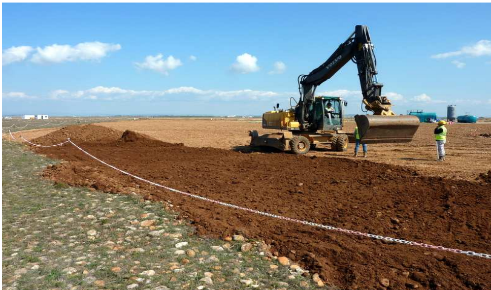
Spreading of the surface layer - RR
