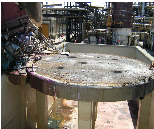
Photos courtesy of DREAL: Concrete base where the tank was positioned
