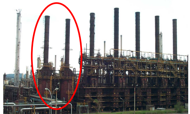
Fig. 2: View of the unit's two superheaters (RR)
