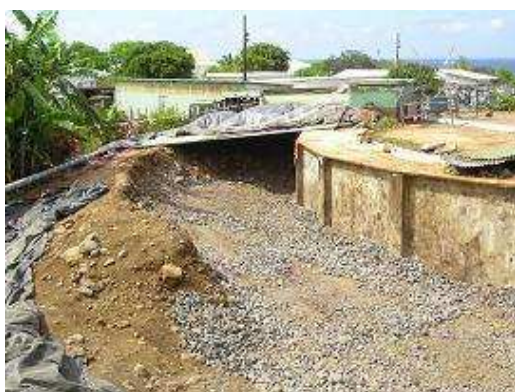
▲ Backfill around tank SEA2 ©
