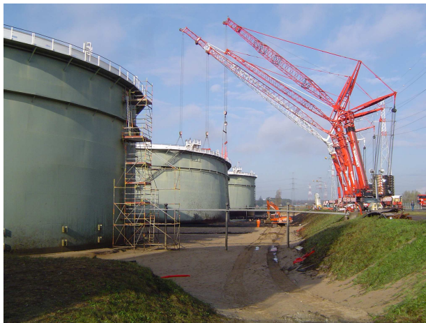
Figure 4: Major cranes stabilising tank D2
