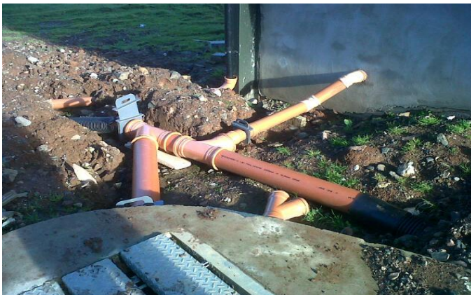
Washing operation of drainage diverter system
