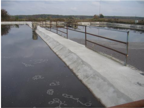
Follow up inspection
