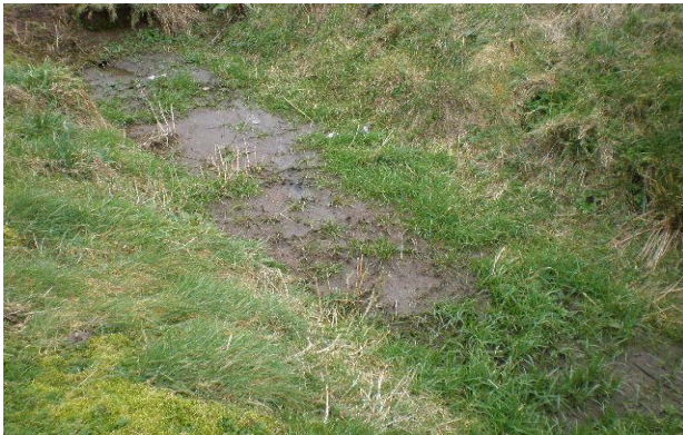
Swale. Contamination due to incorrect diverter setting
