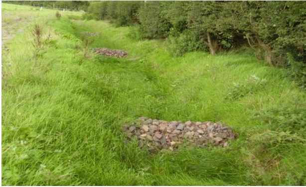
Swale. Treatment of lightly contaminated site run-off
