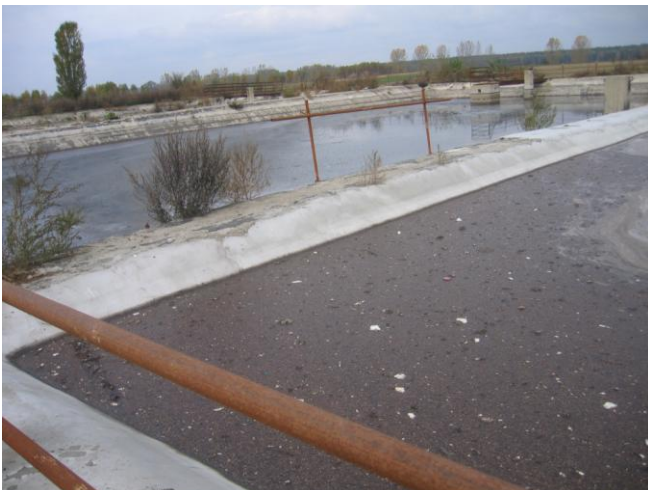
Follow up inspection
