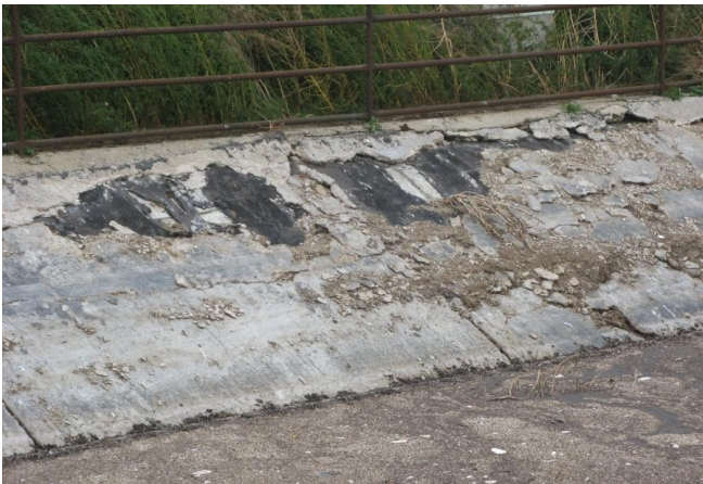
Technical state of the slurry tanks
