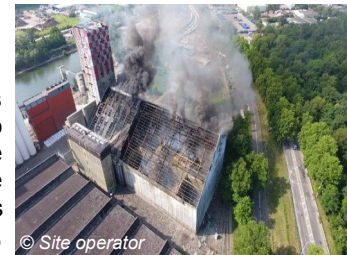
© Site operator Silo explosion linked to inappropriate management of concurrent activities (ARIA 51652)
