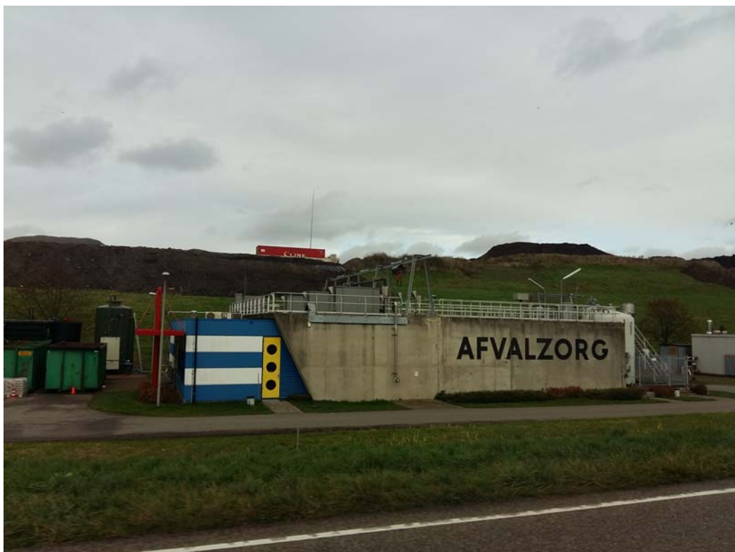
Fig. 8: Wastewater treatment-facility, aerobic treatment
