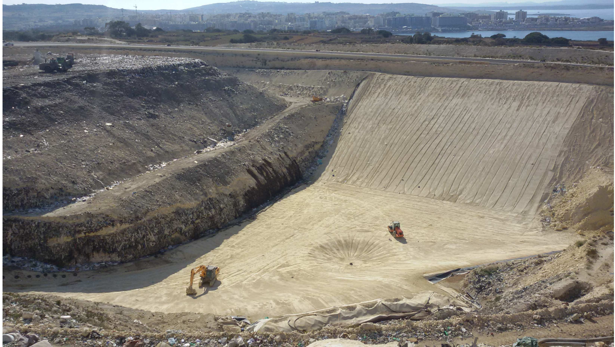
Fig.4: New cell construction
