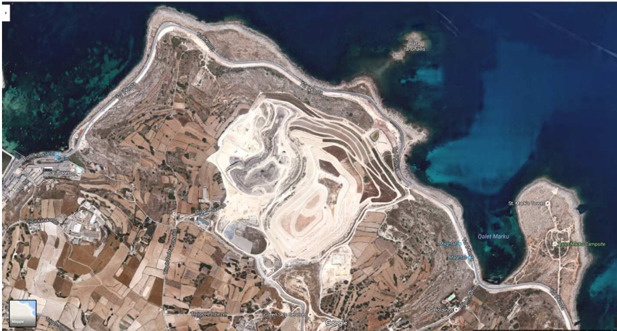
Fig.2: Ghallies landfill view
