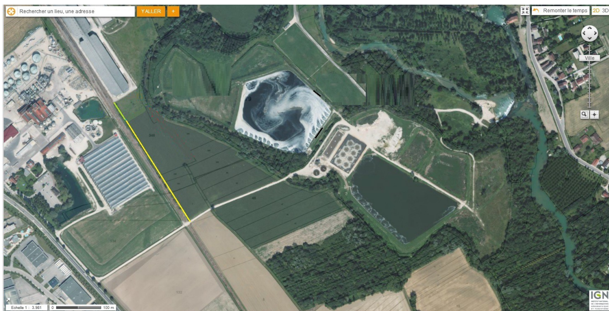
Depiction (in yellow) of the dyke built during this flood episode (ARR operator)
