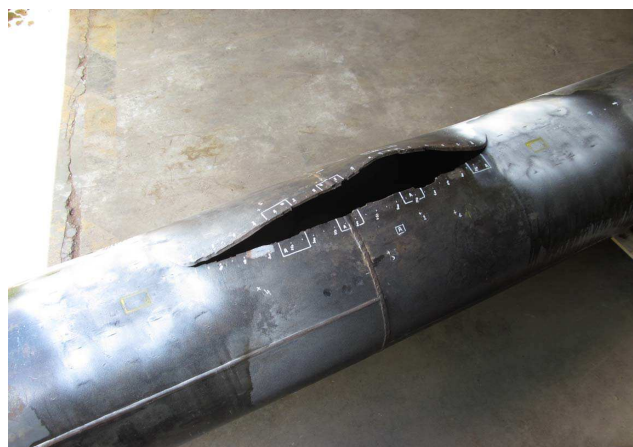
Copyright: Pipeline operator
