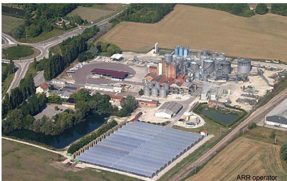
Chemical plant specialised in producing alcohol and recycling solvents, located in Buchères (Aube-10)
