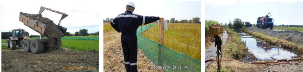
Copyright: Pipeline operator
