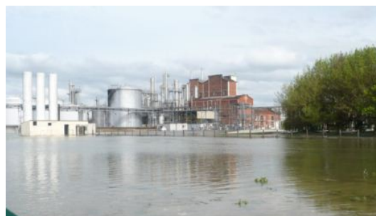
Chemical plant overwhelmed by water (source: DREAL Champagne-Ardenne)
