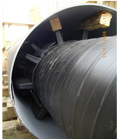
Copyright: Pipeline operator
