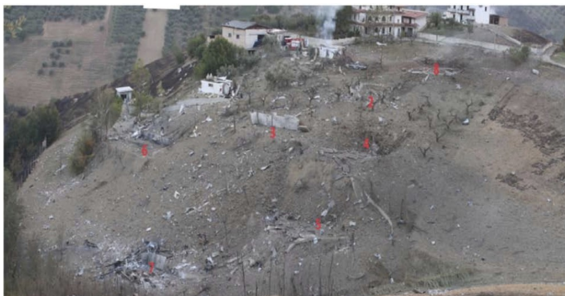
Illustration 2 : The remains of the plant after the accident
