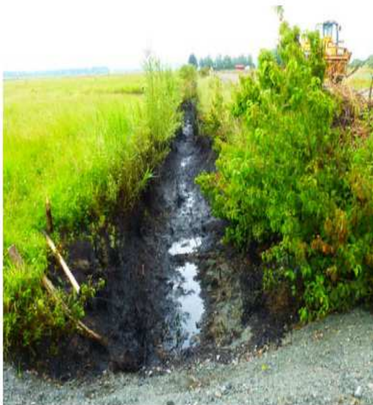
Copyright: Pipeline operator
