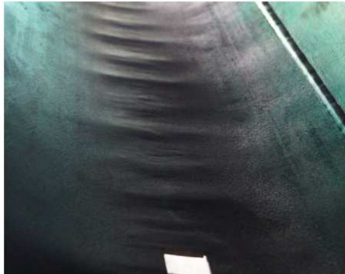
Copyright: Pipeline operator
