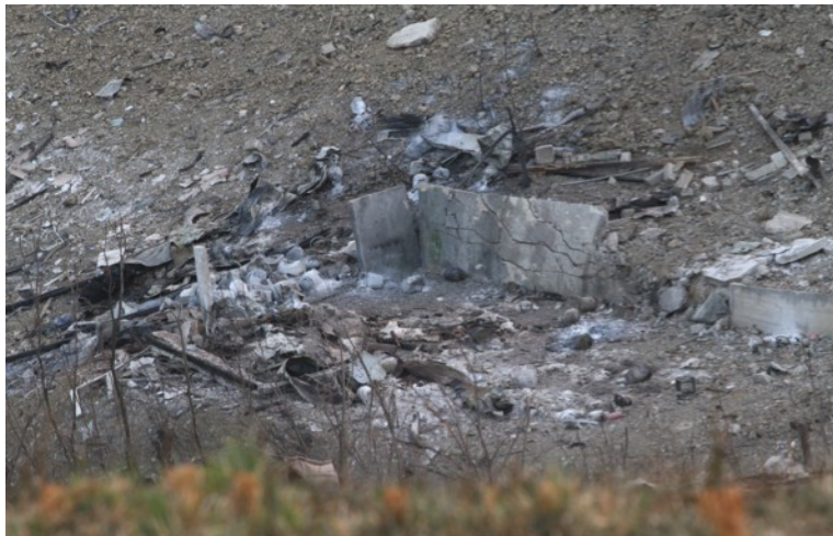
Illustrations 9 and 10 : Damages caused to the buildings and their protection walls
