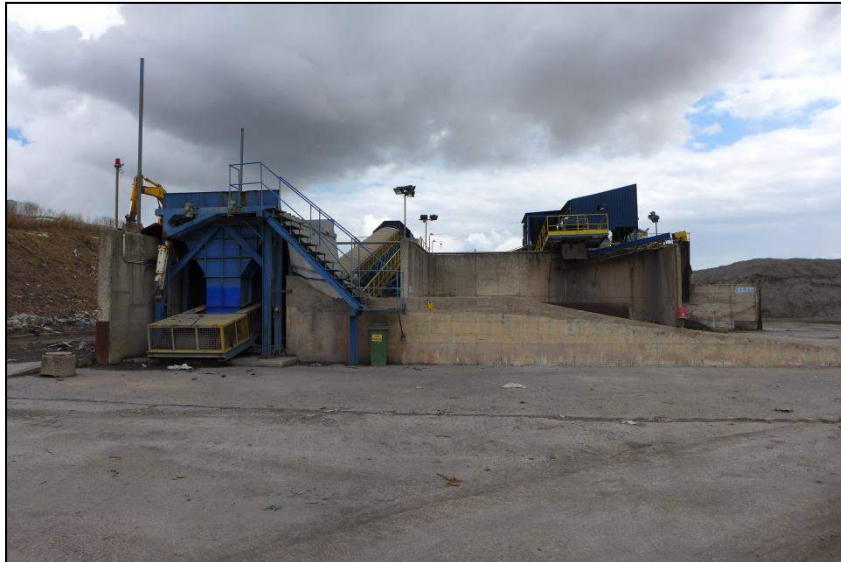
Fig.8: Bottom ash Recovery plant
