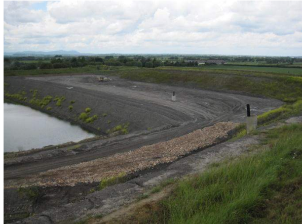
Fig. 10: cell in progress
