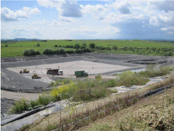
Fig. 9: cell in construction
