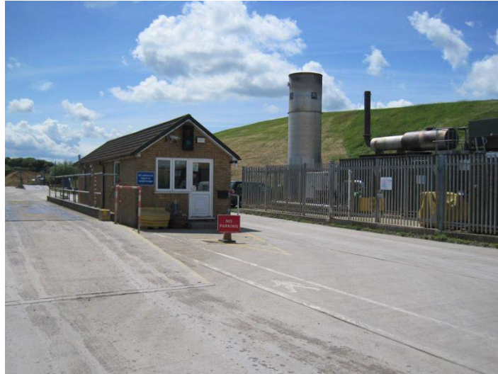
Fig. 8: Landfill gas flare and engine
