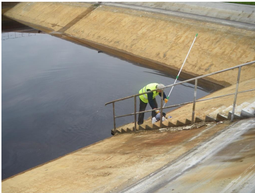
Sampling of leach ate by specialist on sampling of Polish inspectorate
