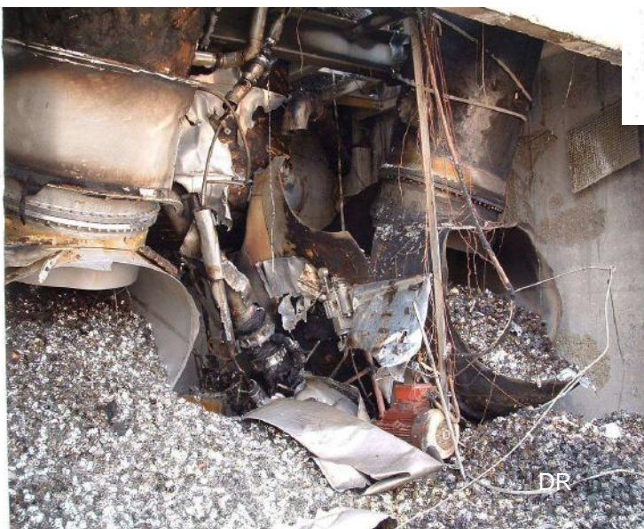
Damaged columns filled with catalyst
