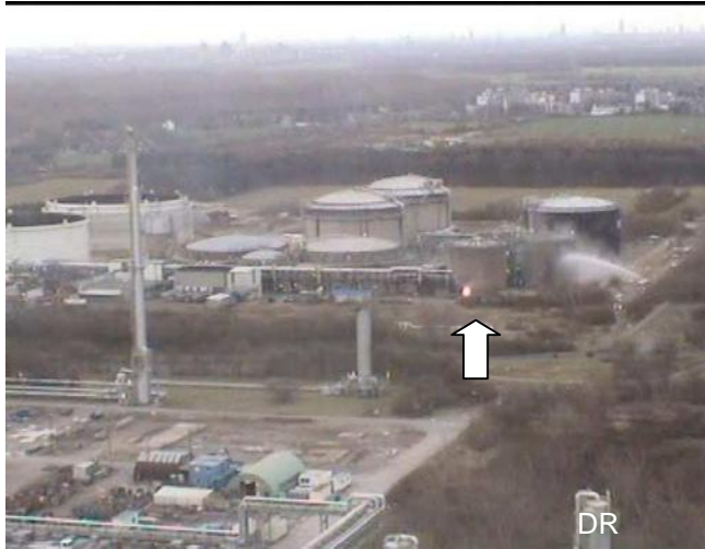
Figure 2: Ethylene flame from the leakage at the insulating flange (arrow) and cooling of the acrylonitrile tanks by the fire brigade
