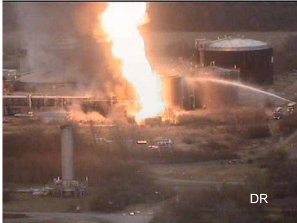
Figure 4: Ethylene jet flame from the broken bypass of the gate valve; gas pressure: 83 bars. Half an hour later the nearest acrylonitrile tank caught fire.
