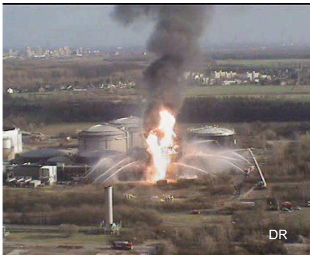
Figure 5: Whole roof area of the acrylonitrile tank is burning at 4:30 pm.
