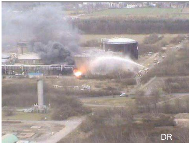
Figure 3: Increasing of the flame in direction of the hydraulic valve and the bypass. Support of the flame by the hot and inflammable hydraulic oil from the broken holding tank of the valve is most likely.
