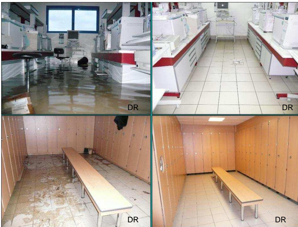
Quick overhaul of facilities (drainage of water, cleaning, drying, tidying up)
