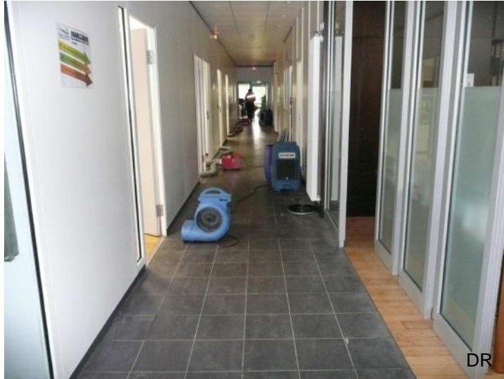
Drying and dehumidification of premises after cleaning and disinfection
