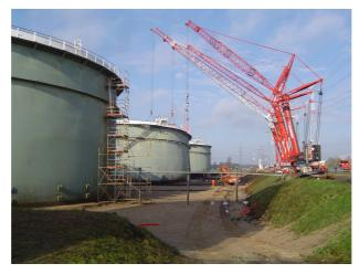
Figure 4: Major cranes stabilising tank D2
