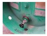
The tank was equipped only with filling and drainage valves and was not equipped with any pressure accessory such as a "pressure gauge" or "safety valve" (see photo).
