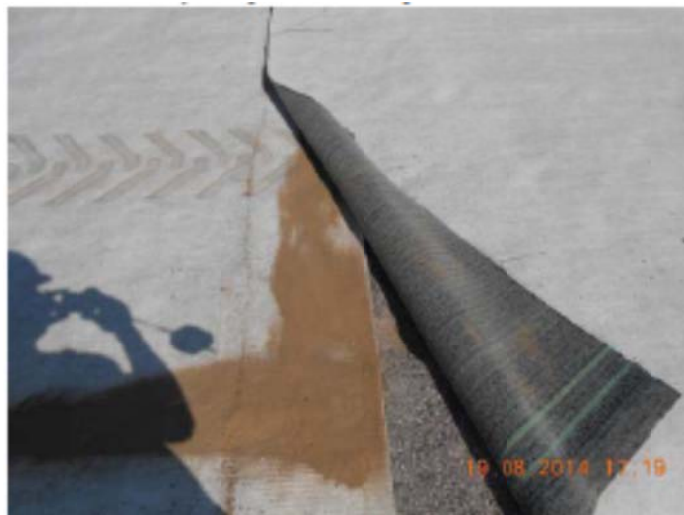
Figure 39: Geosynthetic clay liners
