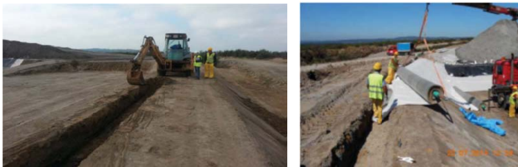
Figure 35: Trenches in coronation slope
