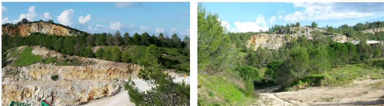
Different perspectives of the rehabilitation going on the Achada e Calhariz Core (Monteiro, C., 2014) 68 .
