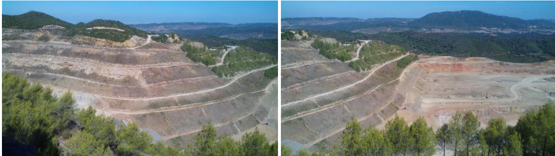
Some aspects of Outão quarries rehabilitation (Correia, A., Ranger on the PNA).
